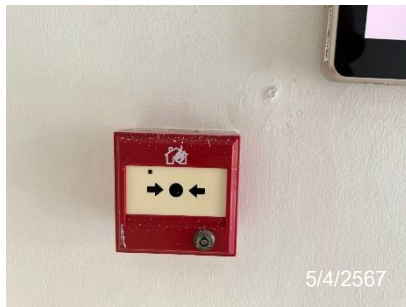
Fire Alarm Manual Station
